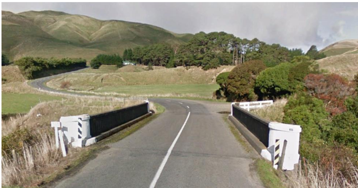
Figure 2.9: Existing bridge on Opaki-Kaiparoro Road
