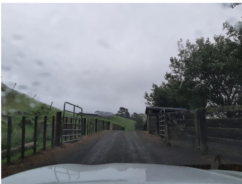
Figure 2.15: Example of a narrow section on Coach Road South, where the road narrows to approximately 3 m
