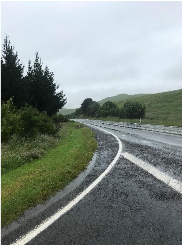
Figure 4.7: Sight distance from Kaiparoro Road, looking north
