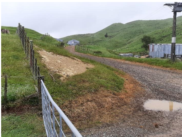
Figure 3.3: Termination of Old Coach Road
