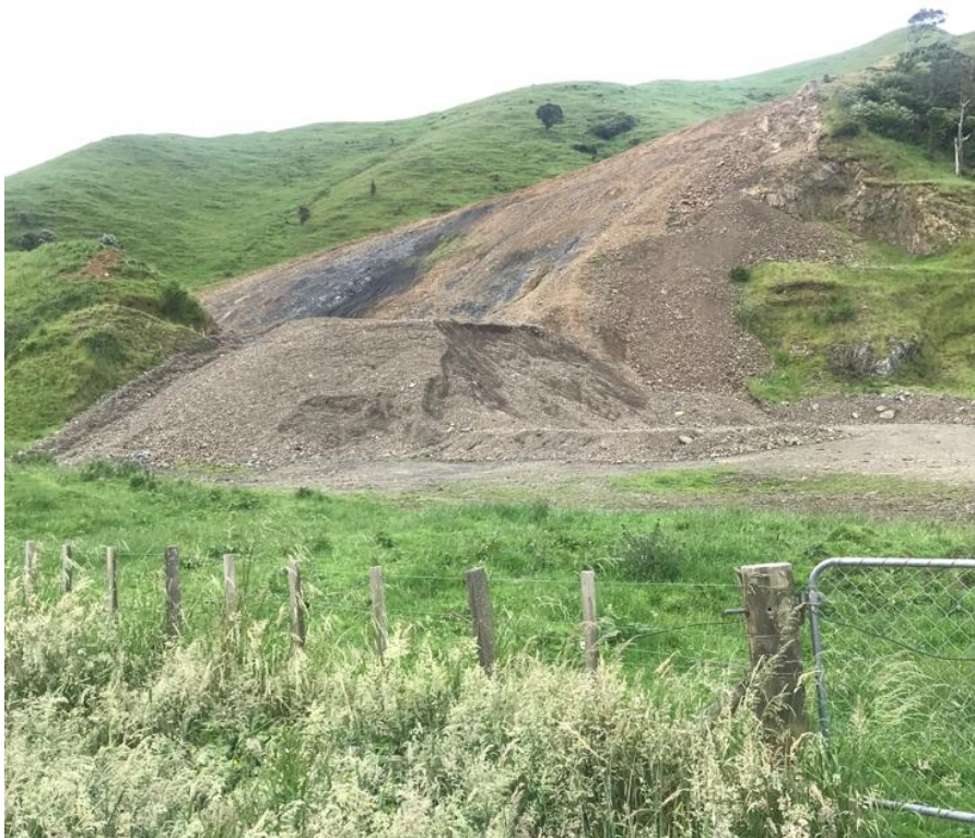
Figure 2.10: Existing quarry on Opaki-Kaiparoro Road
